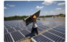
Employees of SunEdison install photovoltaic solar panels on the roof of a Kohl's Department Store in Hillsborough, New Jersey. (Photo by Robert Nickelsberg/Getty Images)
